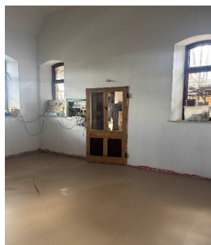
Latex underlay being poured and the new glazing on the internal door
